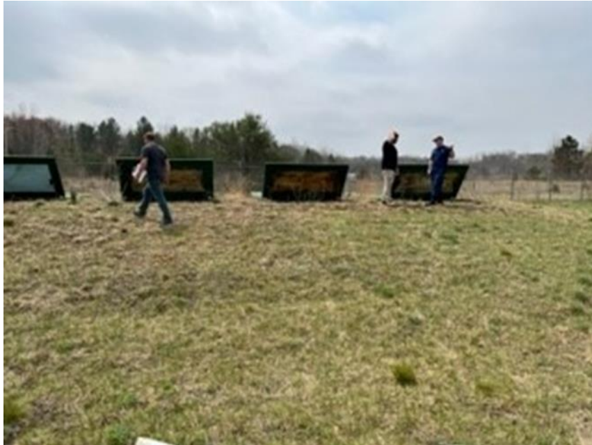
Inspection of Ho-Chunk Che Nunk wastewater treatment site
